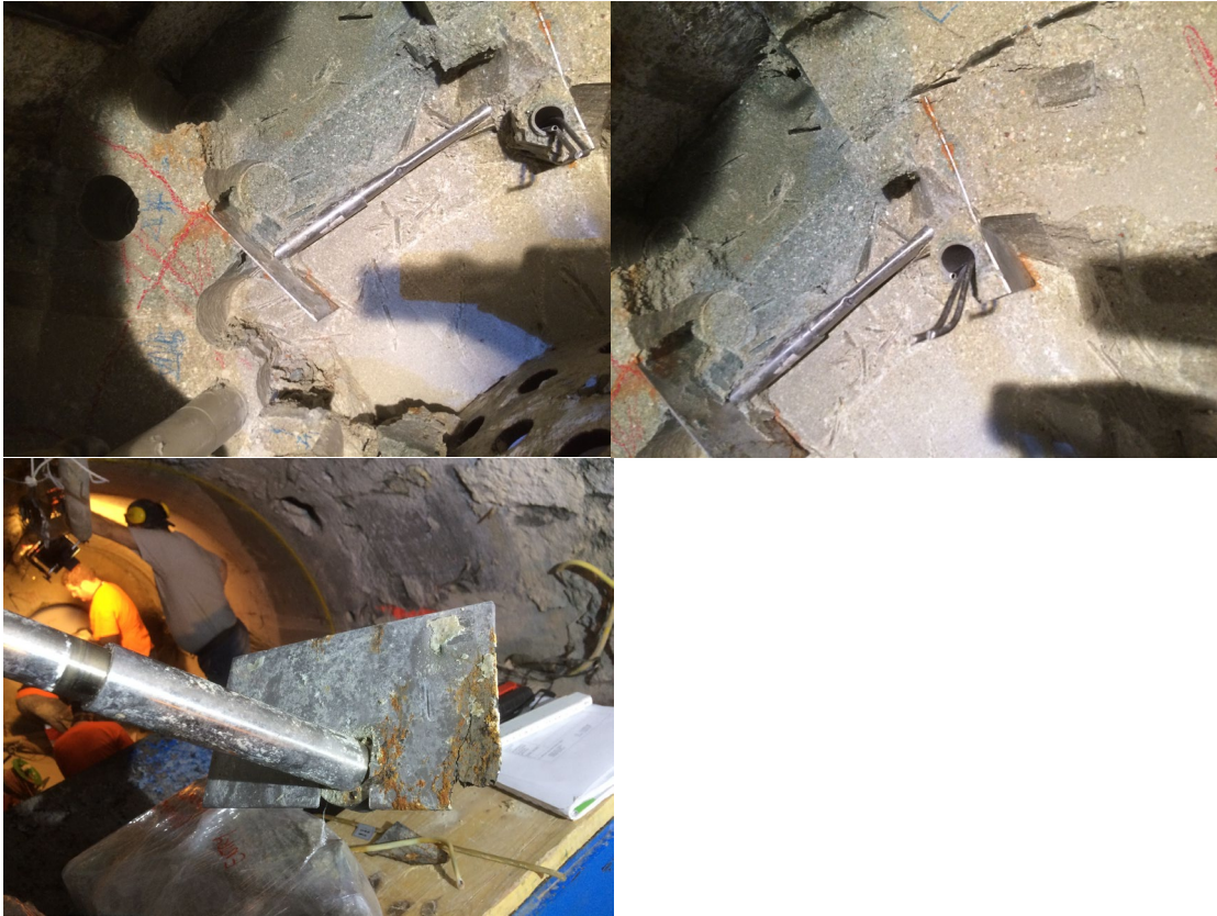
Fig. S48-3: Limited corrosion of extensometer in-between bentonite S-S-48-28/ SBF2-02.
