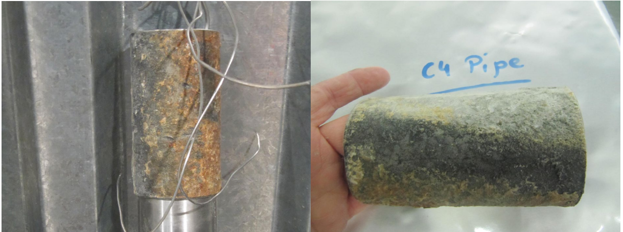
Fig. S42-6: Corrosion features at filters of gas pipes.
