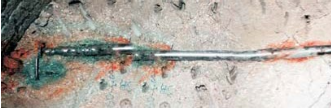
Fig. 4: Extensometer type SH-SD1-01 surrounded by bentonite close to the steel liner (upper left) after dismantling of Heater 1 (from Madina & Azkarate 2004).
