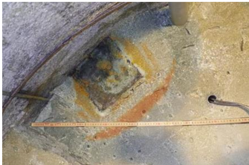
Fig. 57: Picture at top of the fissurometer box after partial removal of bentonite layer 45 in FEBEX-DP project.
