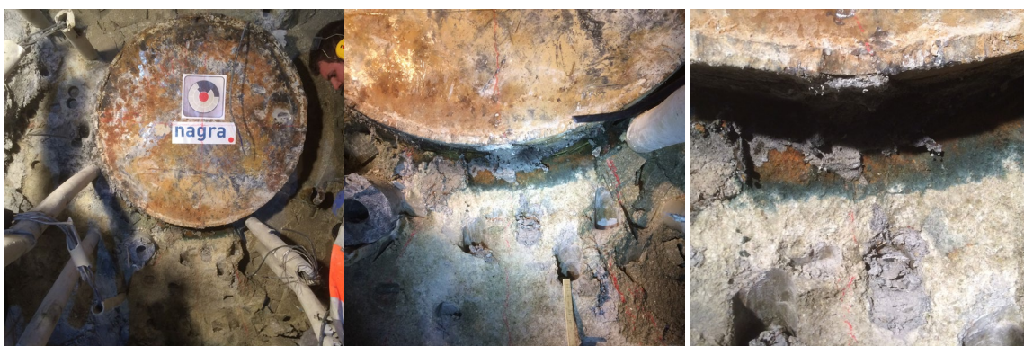
Fig. S36-4: Discoloration zones suggesting various redox conditions around the bottom part of the liner.
