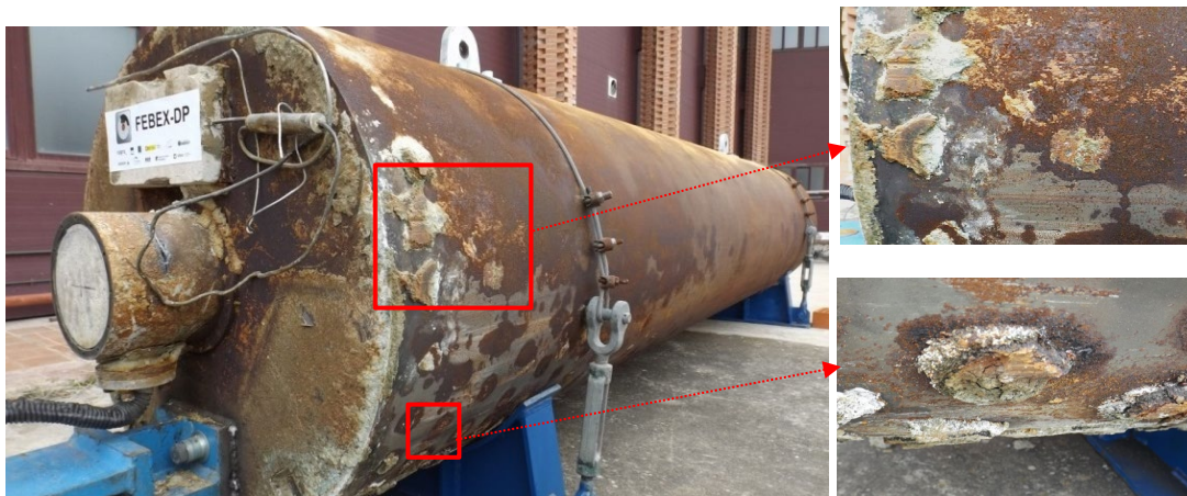
Fig. 23: Heater after transport to AITEMIN facility. Close-up photos showing corrosion features (right).
