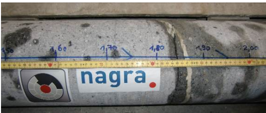
Detail of region at interface between first (on right side) and second plug section, with a sealing layer at 185 cm. Layering from shotcreting is well visible.
