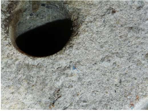
B: Parting surface, without steel fibres, C-C-32-4.
