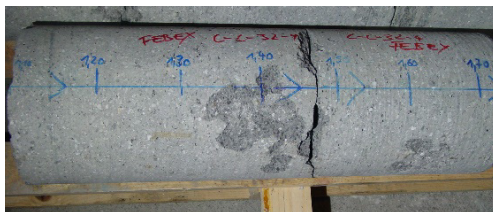
Concrete, second section, 1.1-1.75 m, moist surface
