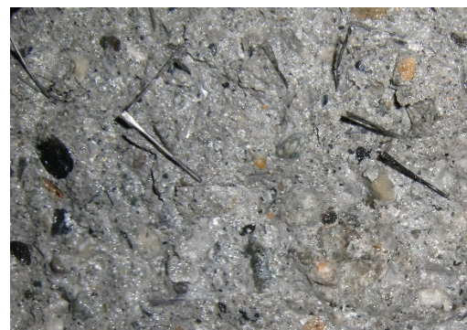
Concrete plug, section with flat-end steel fibres. Wet surface.
